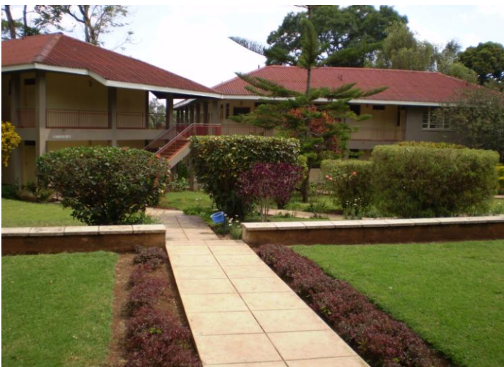
Women's Hostel at Masoka campus
